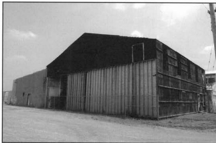
Plating Facility, Louisville
