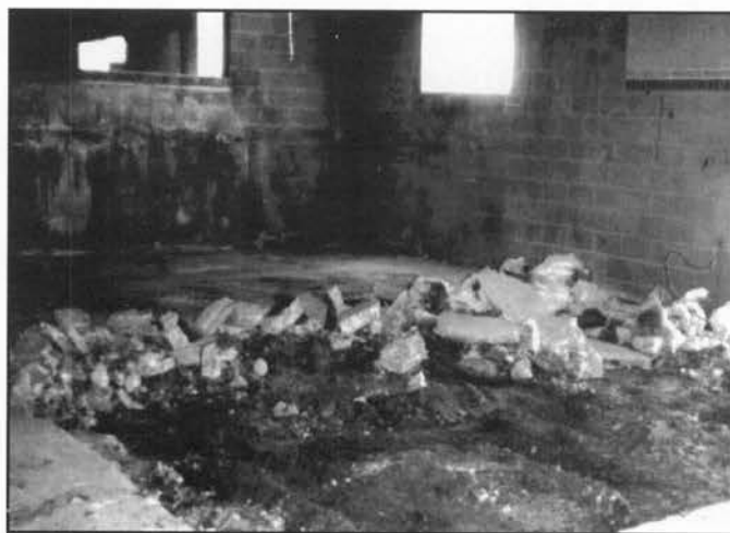
Inside Plating Facility, Louisville
