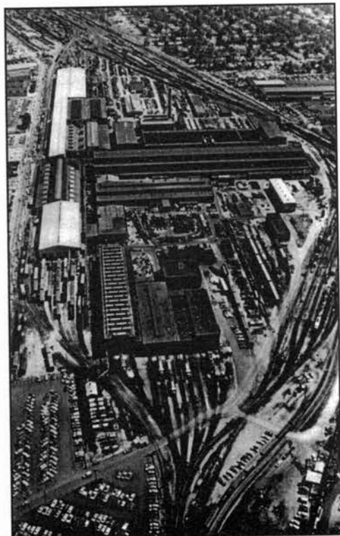
CSX South Louisville Shops at height of operation
