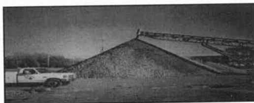
40,000 tons of site foundation crushed and reused
