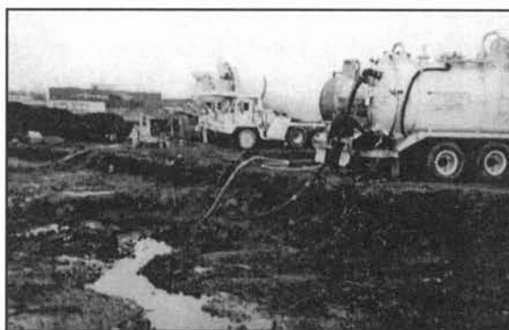
Vacuum Trucks removing diesel fuel during construction
